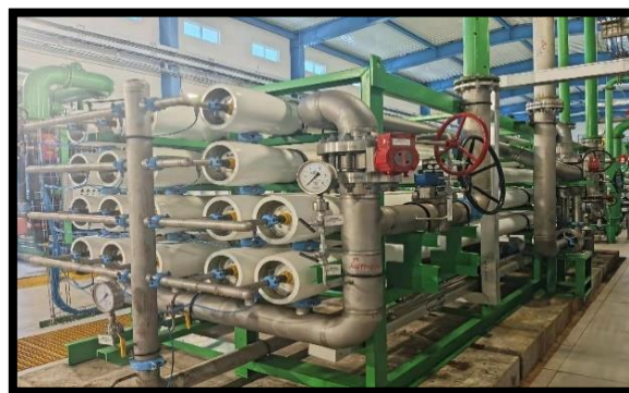
Gambar 1. Tampak depan peralatan SWRO treatment system
