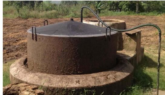
Gambar 2. Tipe digester floating drum
