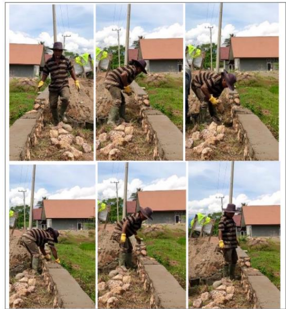
Fig. 1. The positions of field construction workers.
