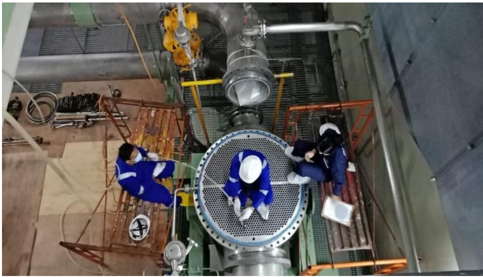
Fig. 6. Nuclear reactor heat exchanger cleaning activities.
