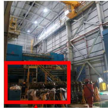
Fig. 5. Implementation combustion inspection on gas turbine GT 2.1.
