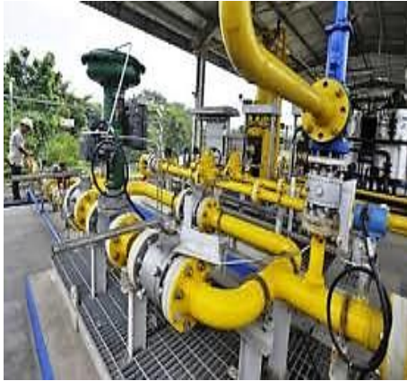
Gambar 3.4 Instalasi Pipa Steam Generator
