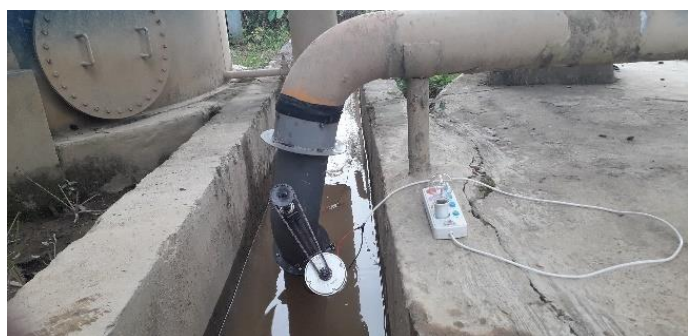
Fig 12. Results of installing a pico-propeller turbine on the PDAM's sewer pipe
