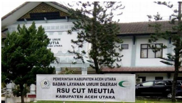
Public Hospital in Lhokseumawe
