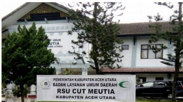
Public Hospital in Lhokseumawe
