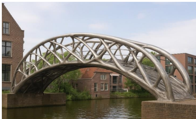
Fig. 4. Illustration of a large structure fabricated by WAAM - stainless steel pedestrian bridge
