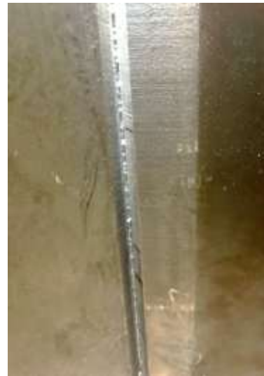
Fig. 4. Welding Seam Before Back Gouging
