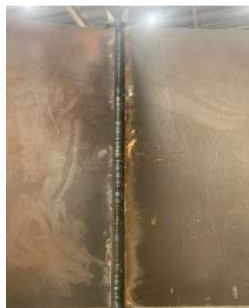
Fig. 5. Welding Seam After Back Gouging Process
