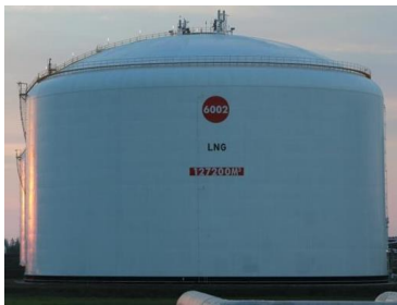
Gbr. 1 Tangki Liquefied Natural Gas (LNG) Storage
