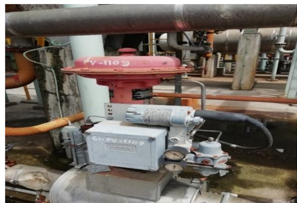
Gambar. 3 Control valve PV1109 (PT Pupuk Iskandar Muda)
