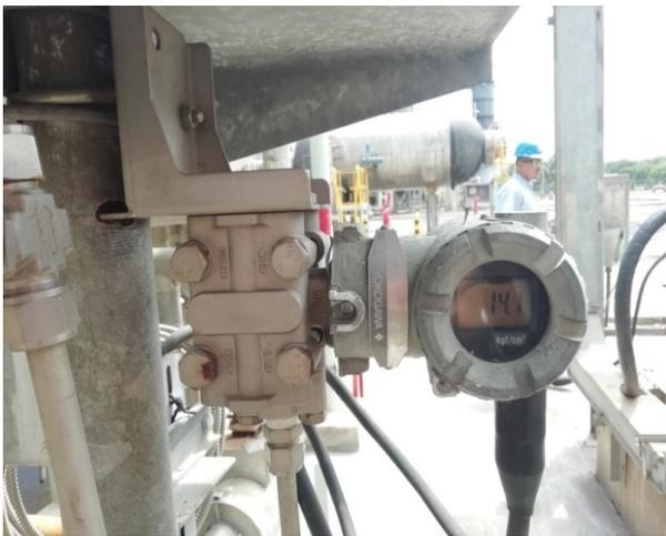
Gambar.3 Pressure Transmitter PT 1109
