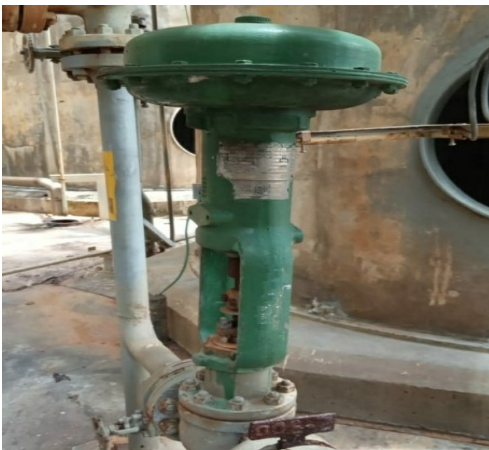
Gambar 4 Globe Valve (PT. Perta Arun Gas)
