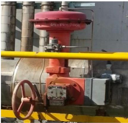
Gambar 3 Control Valve (64 – PV – 7006)
