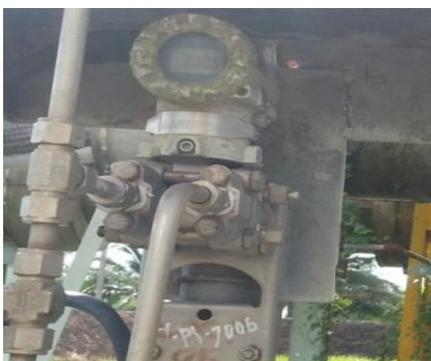
Gambar 4 Pressure Transmitter (64 – PT – 7006)
