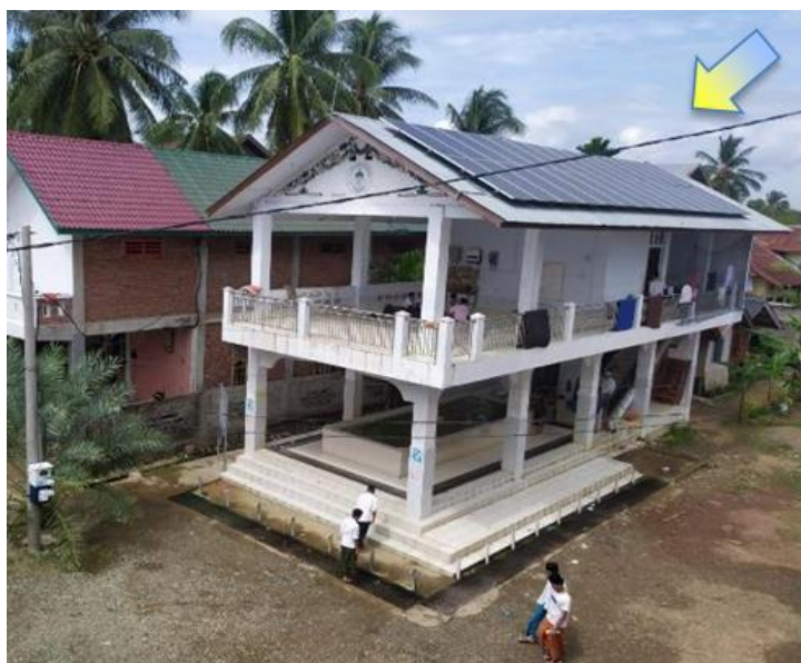
Fig. 4. The position of the rooftop solar panels of Dayah Ulee Titi
